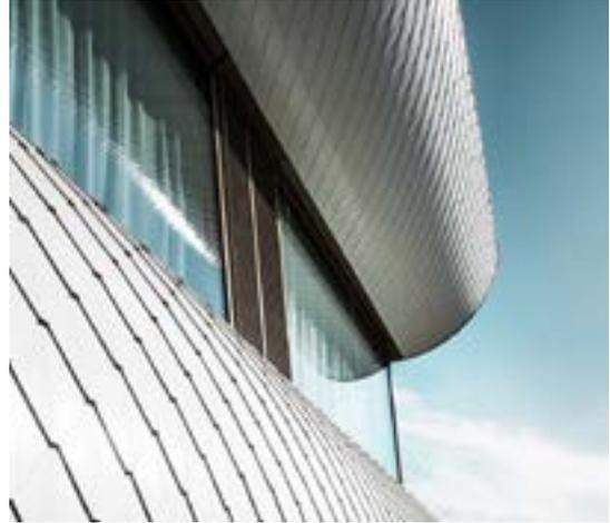
rhomboid panels make the material storm-resistant, they are very light and completely rust-proof since aluminium does not rust. It was a cost-effective realisation of an excellent idea.”
